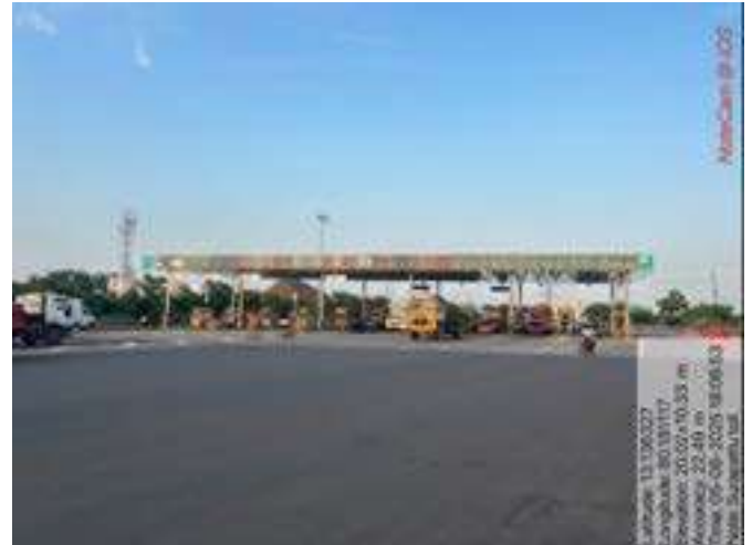
Surapattu Toll Plaza at Km 28+600
