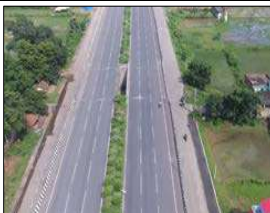
At Grade Separated Junction at Ch. 374+300 RHS
