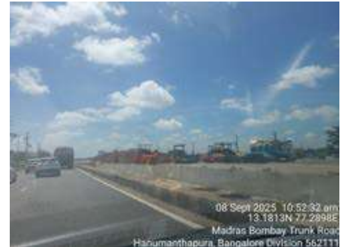
Nelamangala to Dobbaset – Ongoing Construction Activity (6 lanning)
