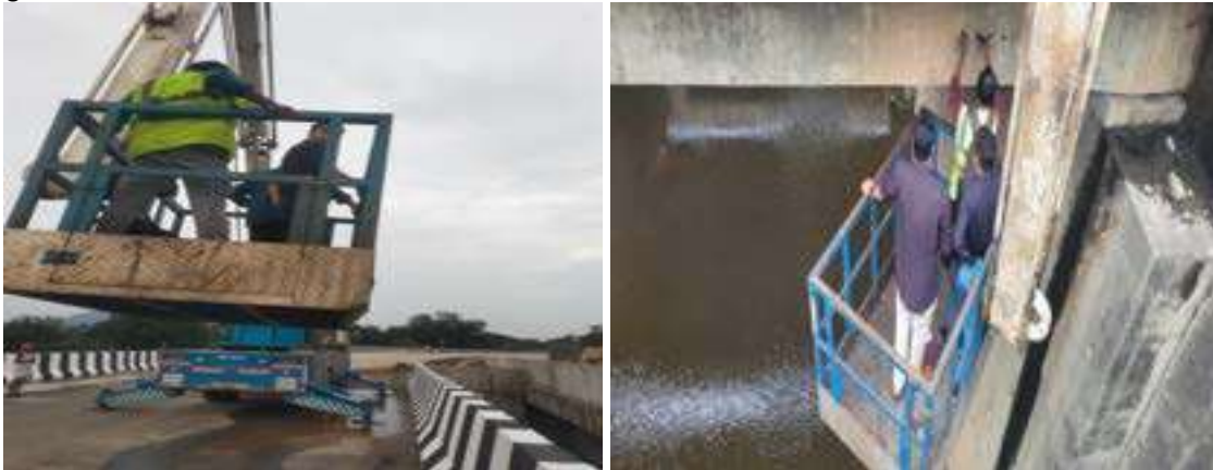
Figure: 3.1 Inspection using MBIU
