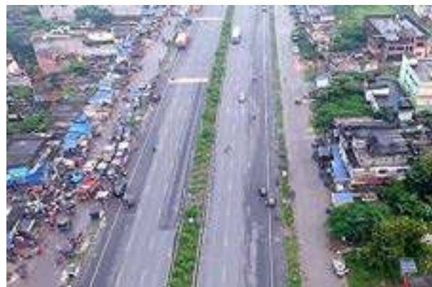
Project Road End at Km 400+632
