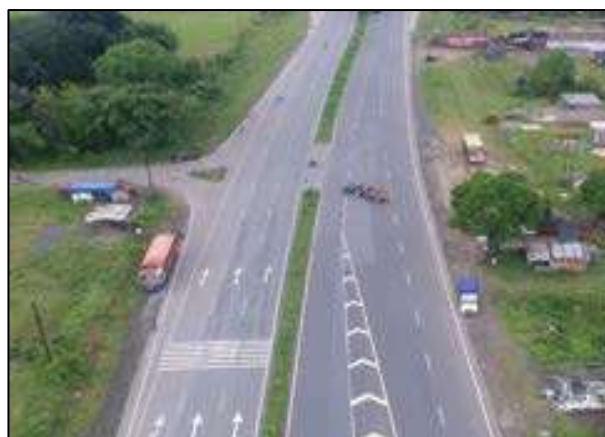
At Grade Junction at Ch. 349+030 LHS
