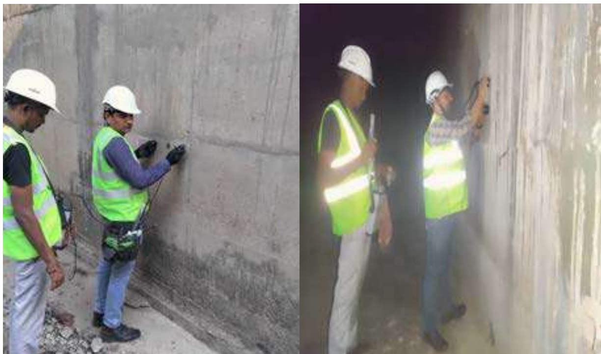
Figure 4.34: Ultrasonic Pulse Velocity Test at Site
