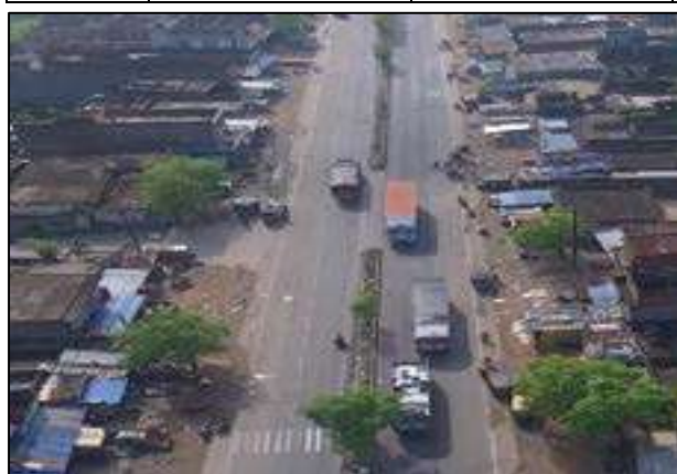
Median Openings at Ch. 323+198
