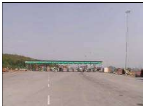
High Mast Light at Toll Plaza 352+100
