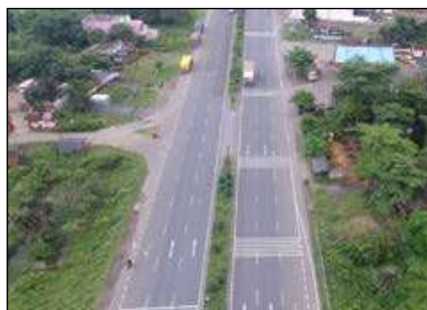
At Grade Junction at Ch. 379+160 LHS
