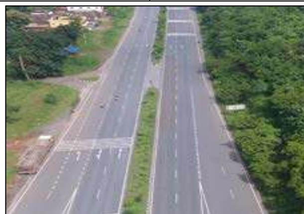
Median Openings at Ch. 371+901
