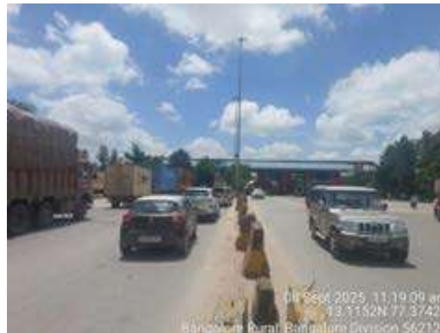
Chokkenahalli Toll Plaza (km 61.470)
