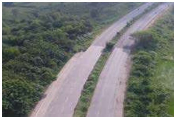
Project Road Start at Km 320+810
