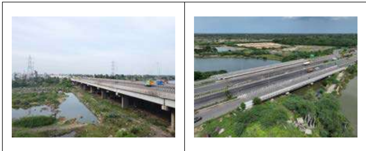
Figure 6-5 : Major Bridges along the Project Stretch
