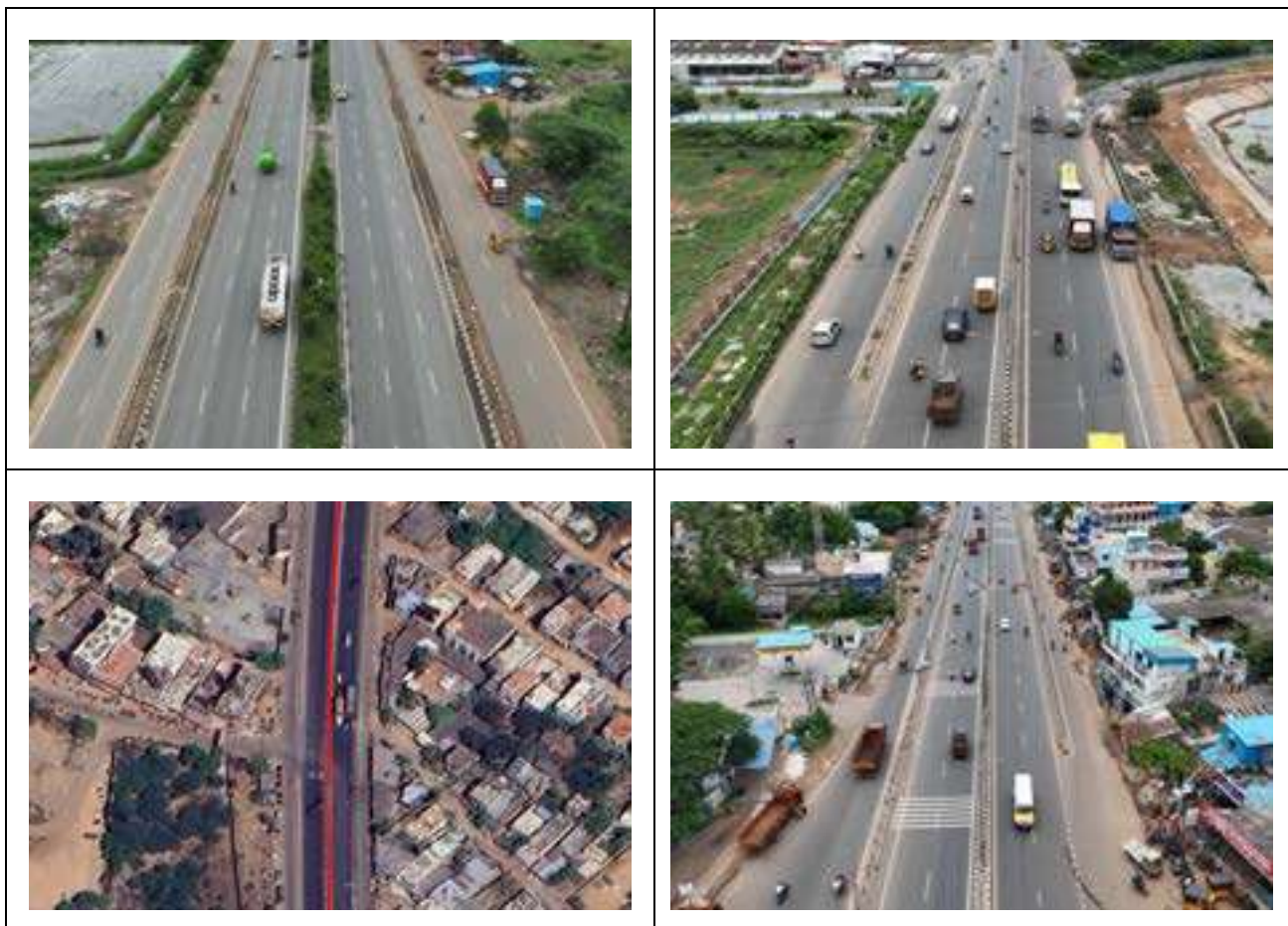
Figure 6-2 : Service Road along the Project Stretch
