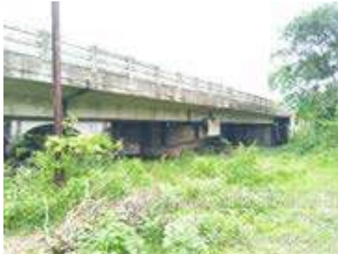
Minor Bridge at Km 348+112
