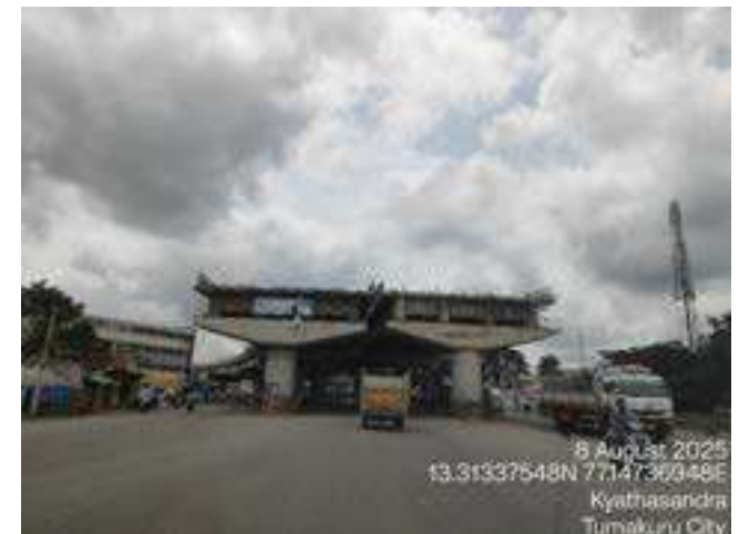
Tumakuru Bypass – ongoing 4 to 6 lane construction activities
