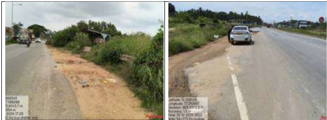
Figure 6-7 : Bus Bay along the Project Stretch
