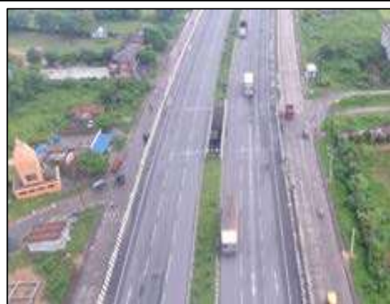
At Grade Separated Junction at Ch. 395+750 RHS
