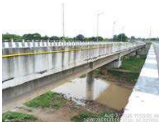
MAJOR BRIDGE AT Km 333+330
