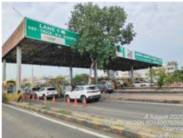
Vanagaram Toll Plaza (km 16.620)
