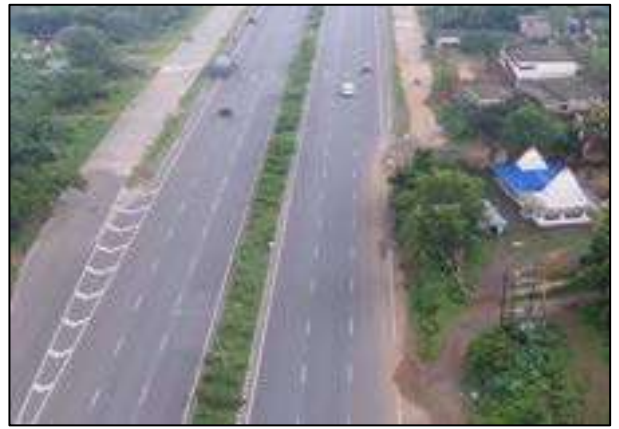
Temple at Ch. 382+390 RHS Service Road
