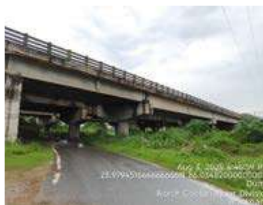
MAJOR BRIDGE AT Km 357+418
