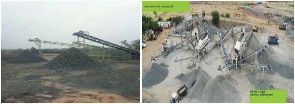
Photographs of Aggregate source at Km 400+132
