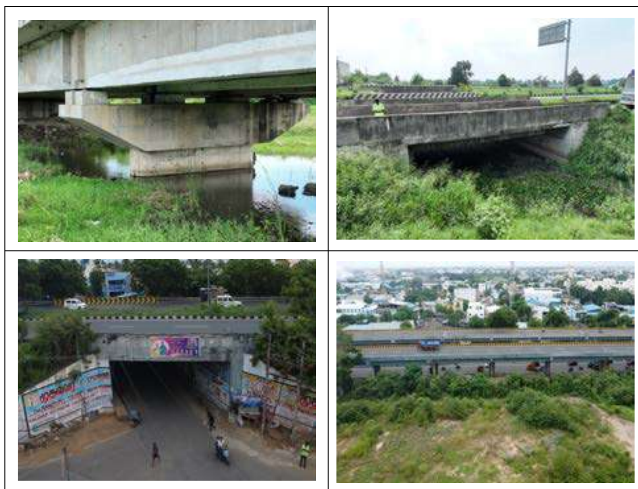
Figure 3-6: Inventory and Condition Surveys of Existing Structures
