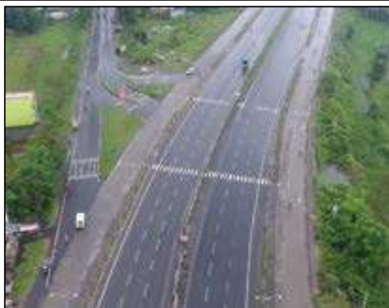
At Grade Junction at Ch. 353+950 LHS
