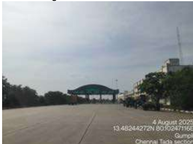
Modern Integrated Check Post
