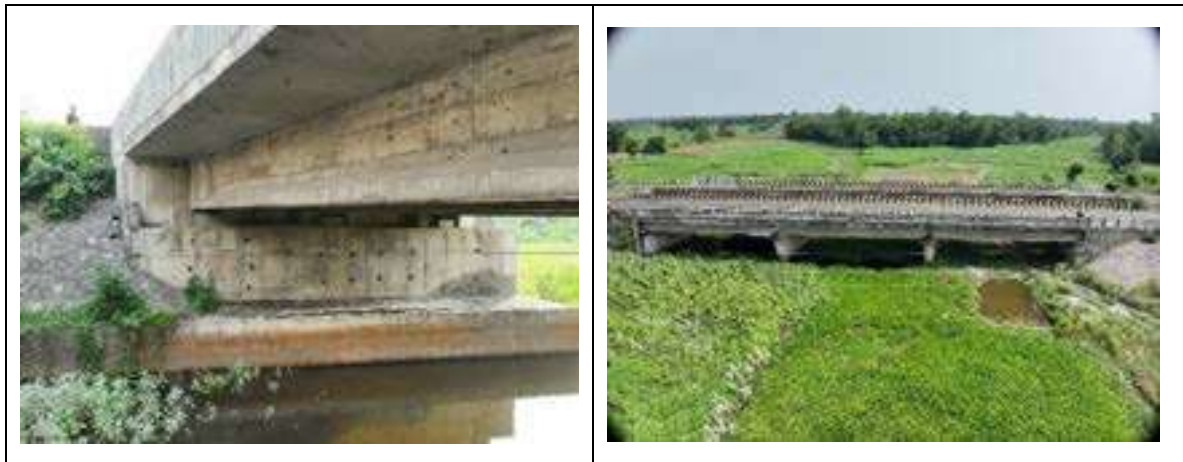
Figure 6-6 : Minor Bridges along the Project Stretch
