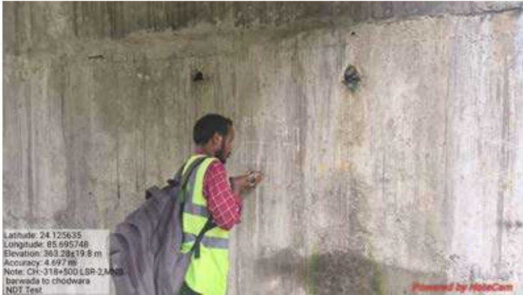
Figure: 3.2 Rebound Hammer Test
