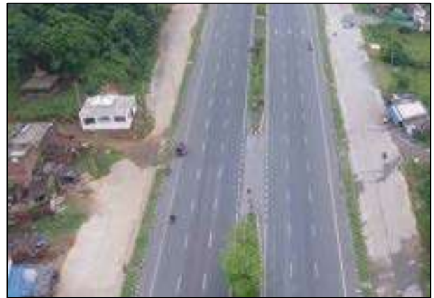
Temple at Ch. 361+050 LHS Service Road
