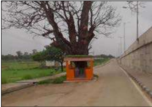
Temple at Ch. 339+120 RHS Service Road
