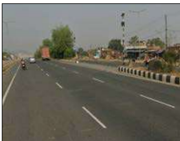
Traffic Blinkers Light at 361+038
