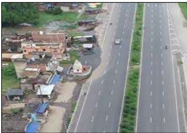
Temple at Ch. 368+935 LHS Service Road
