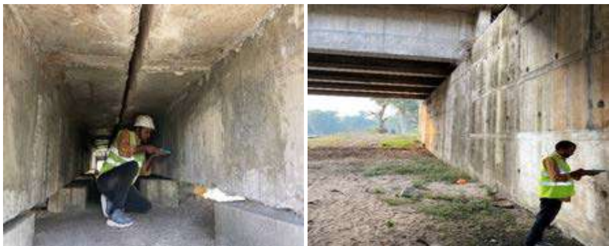
Figure 4.31: Rebound Hammer Test at Site
