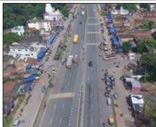
At Grade Junction at Ch. 375+850 RHS
