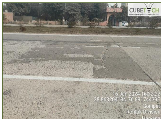
Figure: Tranverse Cracks
