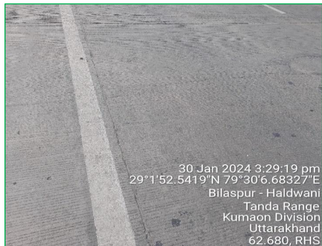
Figure 0-2: Tranverse Cracks
