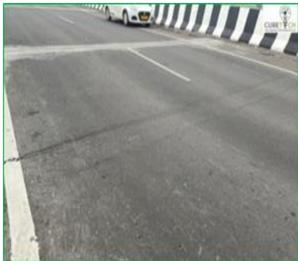
Figure 7-6: Transverse cracks
