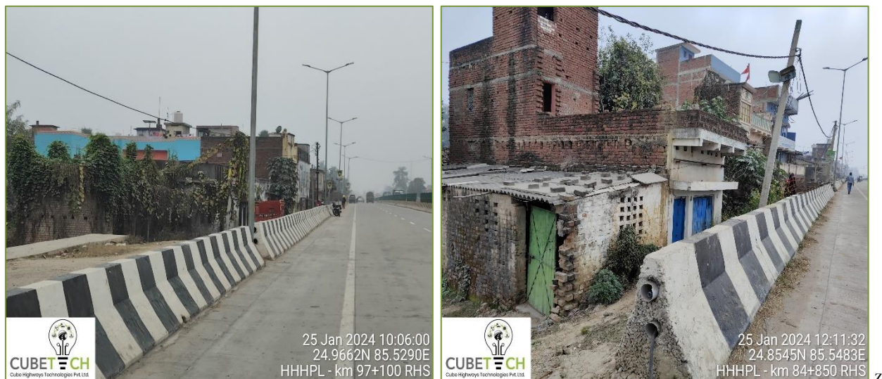
Figure 3-7: Rigid Crash Barrier
