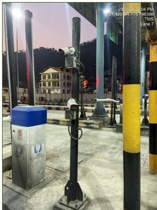
Figure 3-14: LPIC and ICS Cameras
