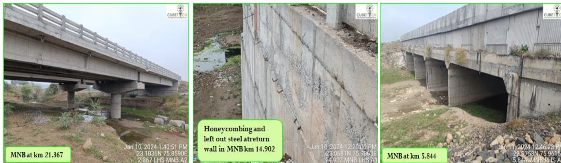
Figure 4-2: Condition of Minor Bridges
