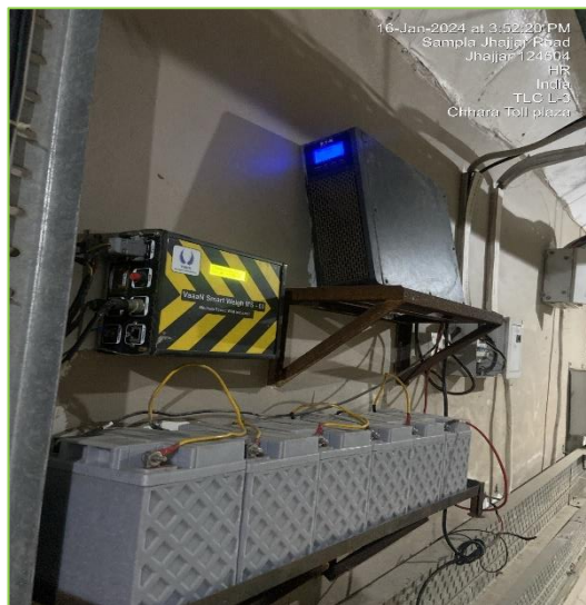
Figure 3-23: Lane UPS in Tunnel.
