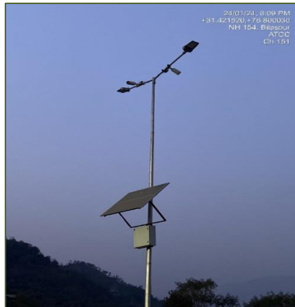
Figure 3-27: Camera Based ATCC.
