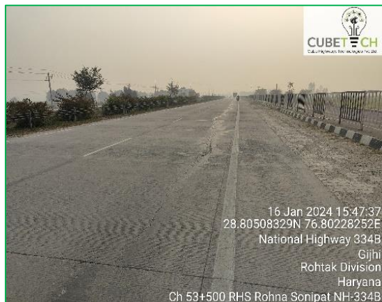
Figure: Longitudinal Cracks
