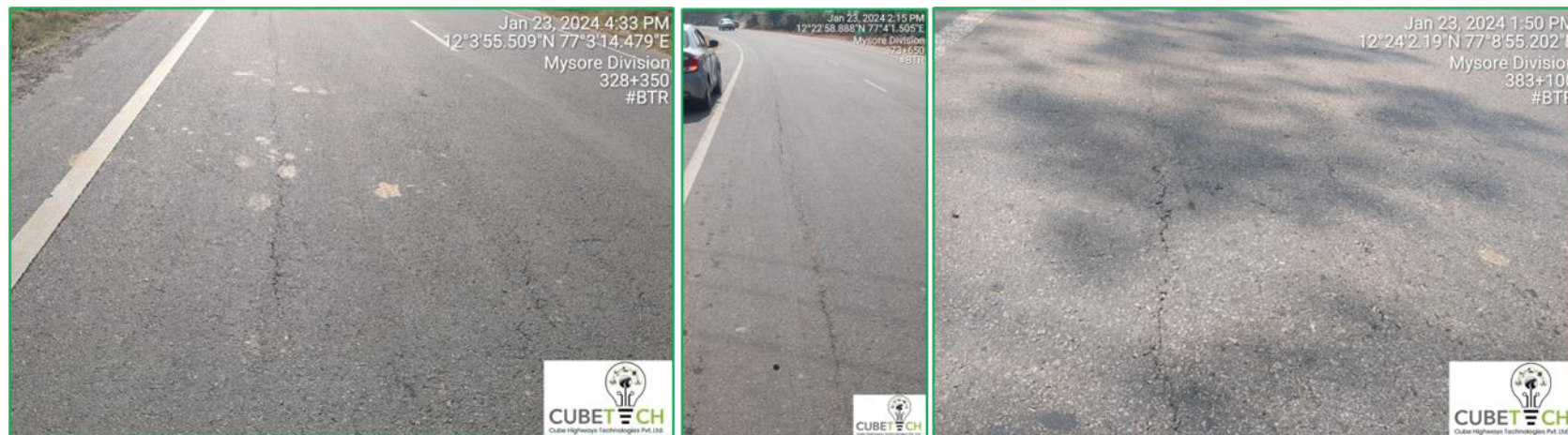
Figure 7-6: Longitudinal Cracks
