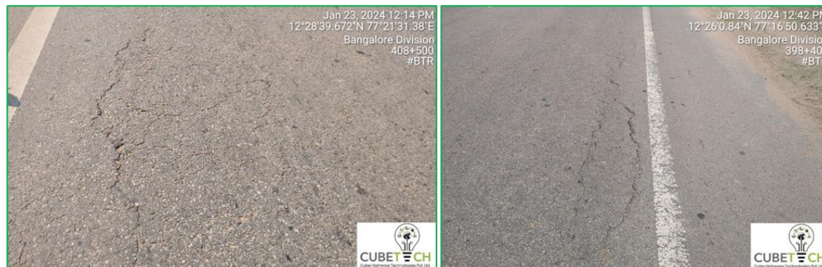
Figure 7-7: Alligator Cracks
