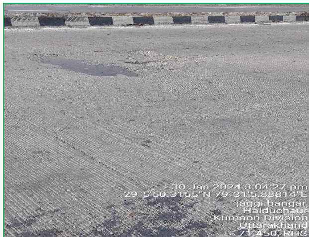
Figure: Scaling
