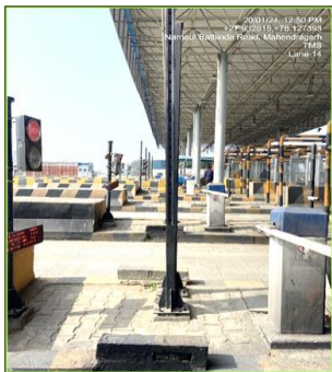
Figure 3-10: AVC Height Sensors
