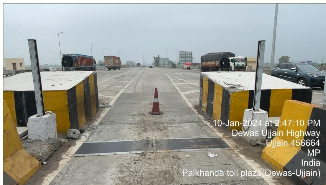
Figure 3-22: Medium Speed Weigh in Motion (MSWIM)
