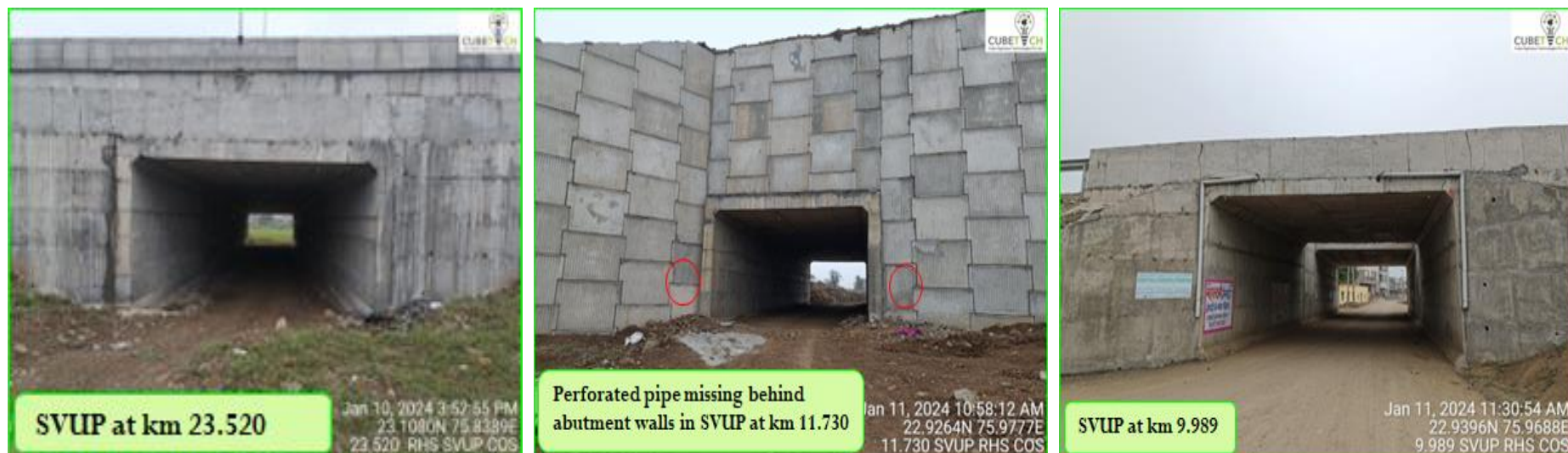
Figure 4-7: Condition of LVUPs
