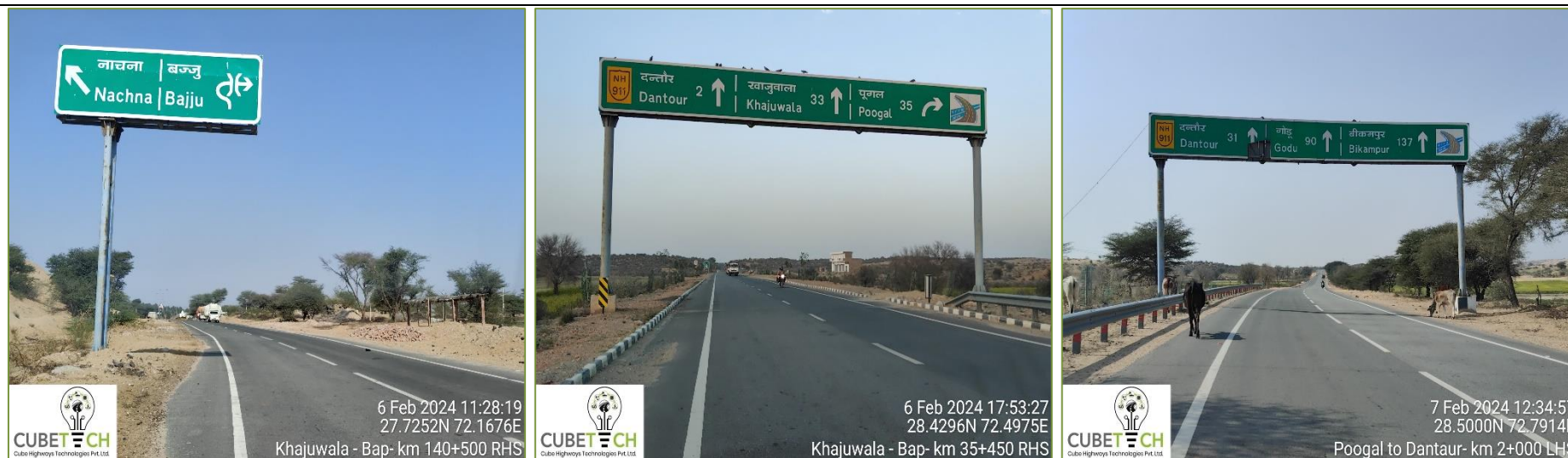
Figure 3-6: Overhead & Cantilever Gantry boards
