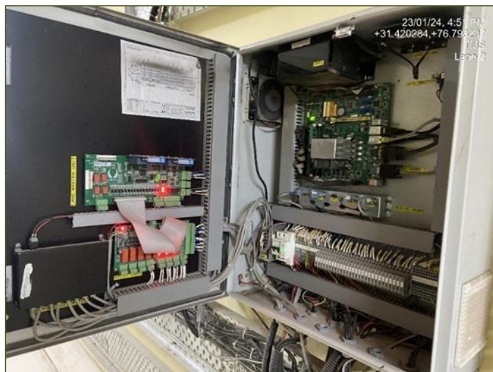
Figure 3-10: Toll Lane Controller inside Tunnel.
