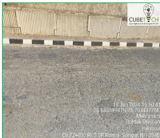
Figure: Alligator Cracks
