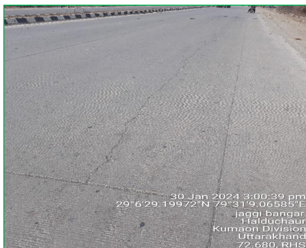
Figure 0-1: Longitudinal Cracks
