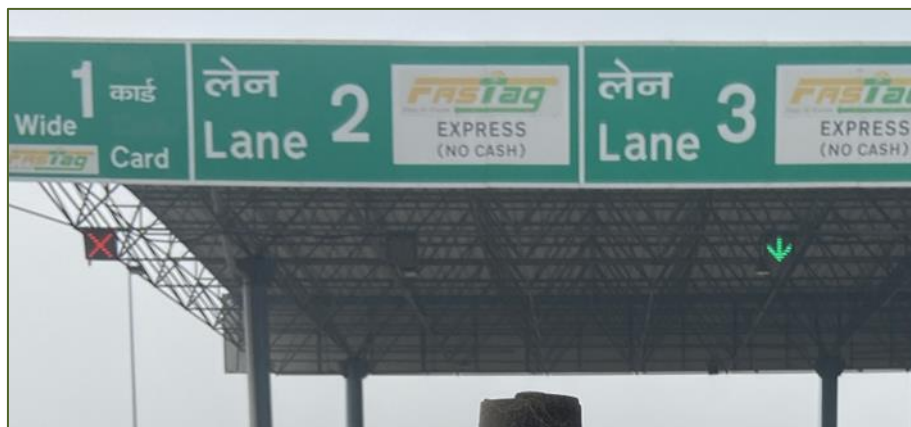
Figure 3-15: Over Head Lane Signal (OHLS).
