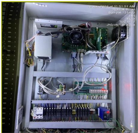
Figure 3-9: Toll Lane Controller at Tunnel
