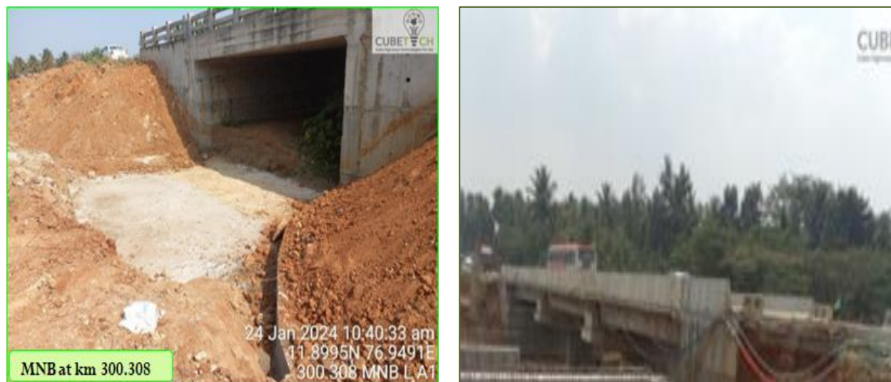
Figure 4-2: Condition of Minor Bridges at km 300+308 & 443+075
