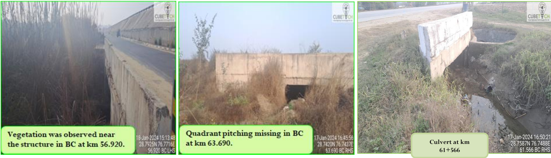
Figure 4-6: Condition of Culverts
