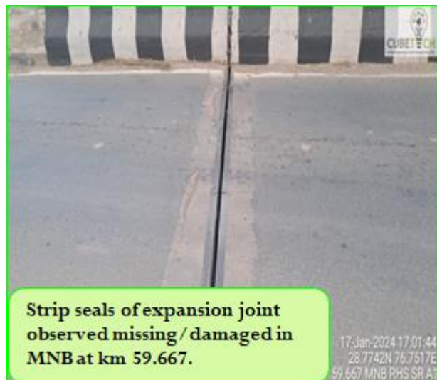
Figure 4-1: Condition of Minor Bridges
