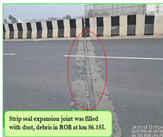
Figure 4-2: Condition of Road Over Bridges
