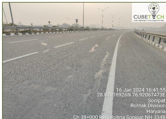
Figure: Longitudinal Cracks
