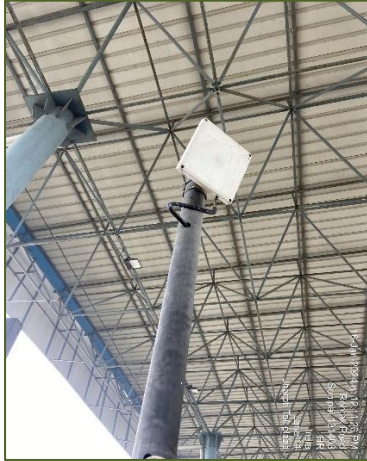
Figure 3-8: RFID reader.
