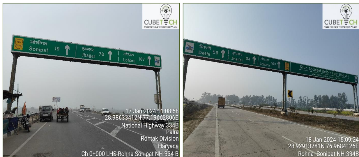
Figure 3-5: Overhead & Cantilever Gantry boards and VMS
