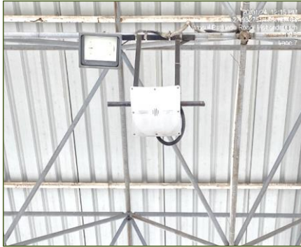
Figure 3-8: RFID Reader.
