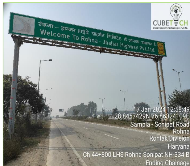
Figure 3-5: Overhead & Cantilever Gantry boards
