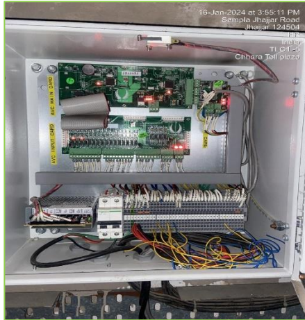
Figure 3-12: AVC enclosure.
