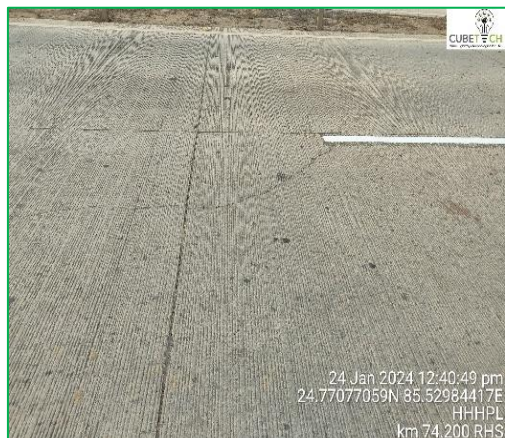
Figure: Corner Break
