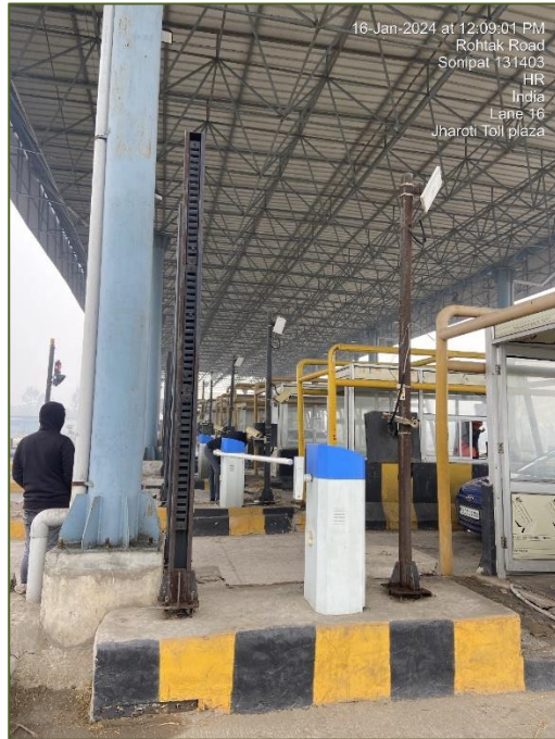
Figure 3-11: AVC IR Sensor.
