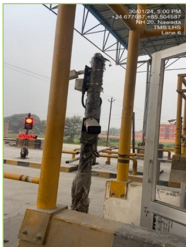
Figure 3-20: LPIC and ICS Cameras.
