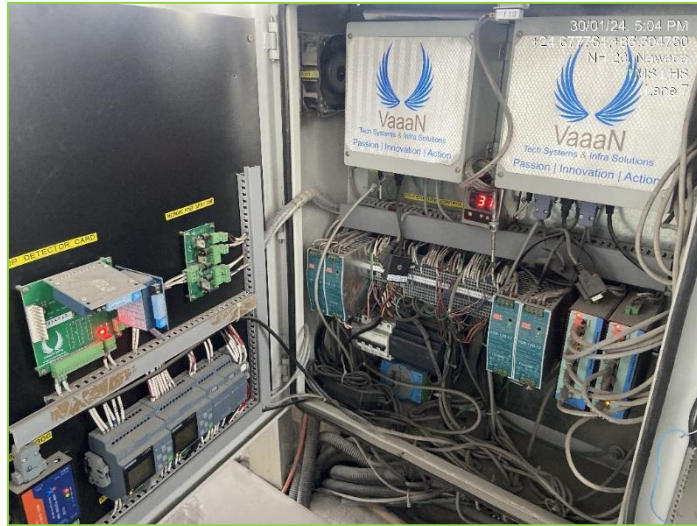
Figure 3-16: Toll Lane Controller inside Booth
