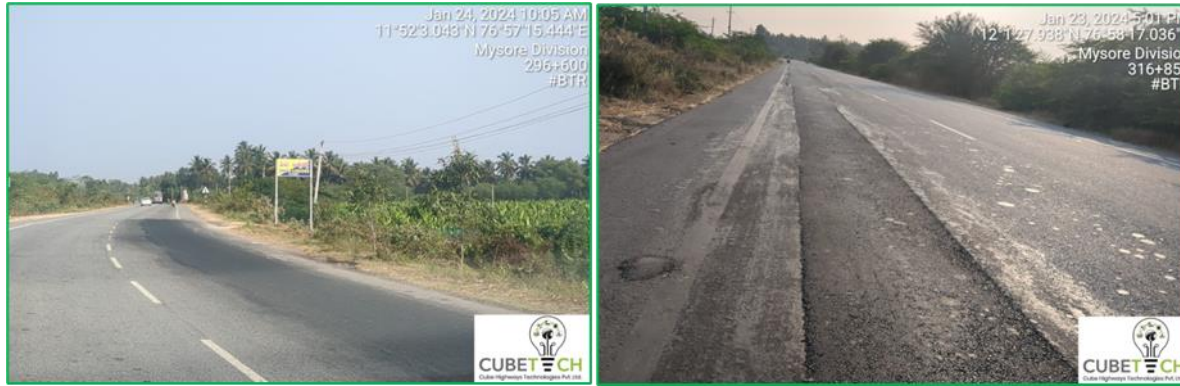
Figure 7-11: Patches
