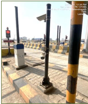
Figure 3-13: LPIC and ICS Cameras.
