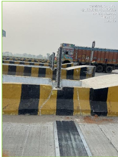
Figure 3-23: Medium Speed Weigh in Motion (MSWIM).
