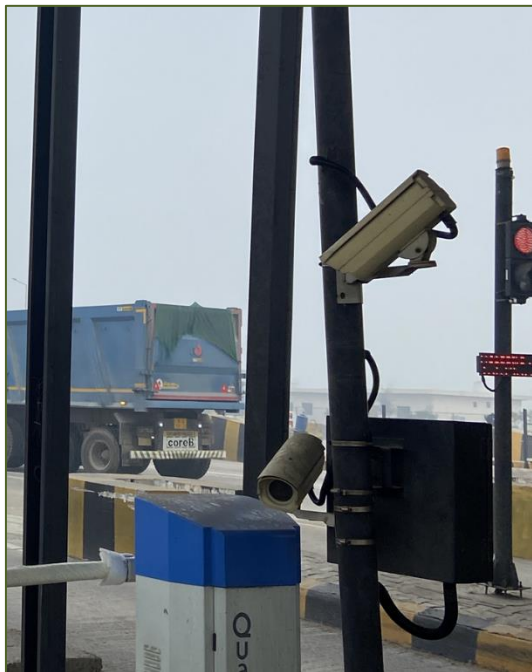
Figure 3-14: LPIC and ICS Cameras.
