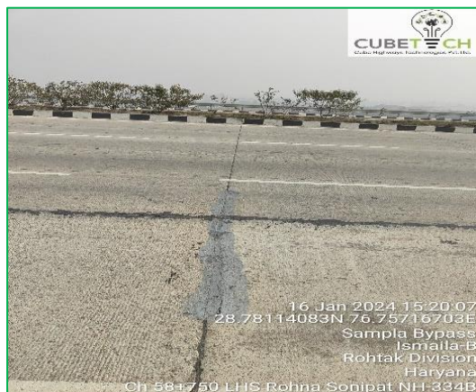
Figure: Spalling of joints
