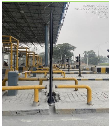
Figure 3-17: AVC Profiler.
