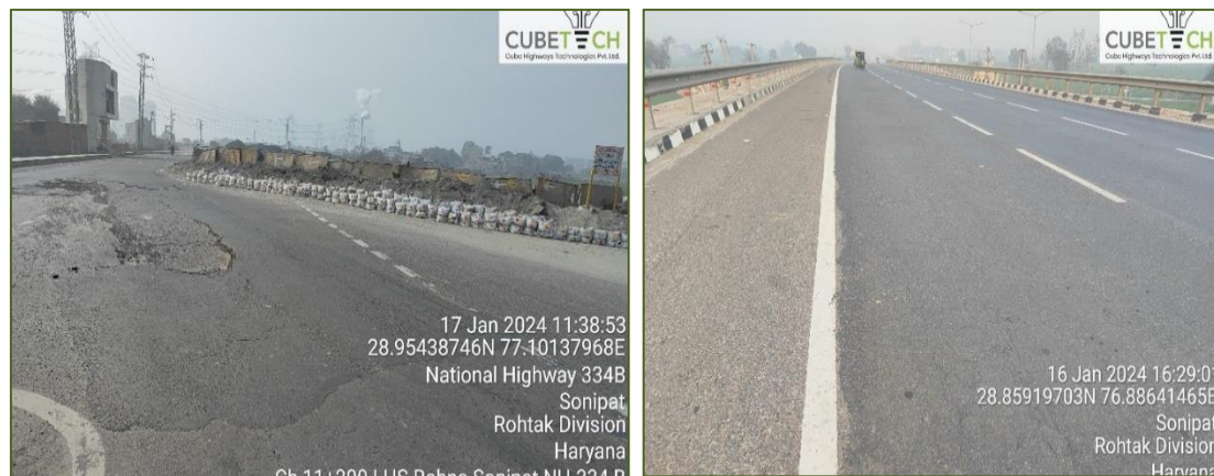
Figure: Alligator Cracks
