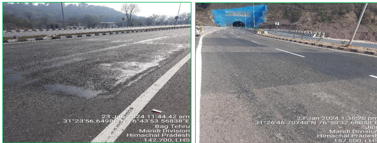
Figure: Patches
