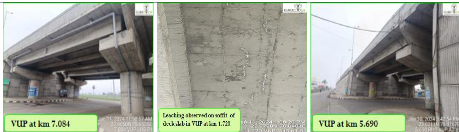
Figure 4-5: Condition of VUPs
