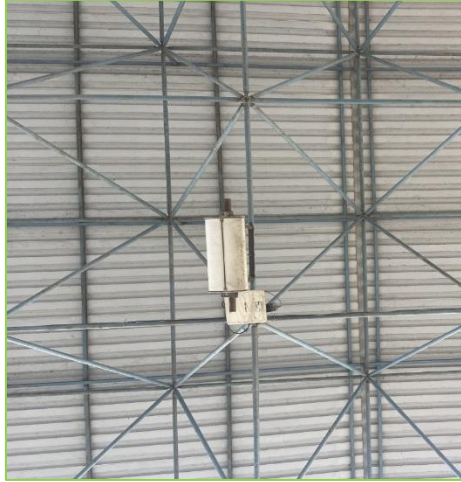
Figure 3-9: RFID reader.
