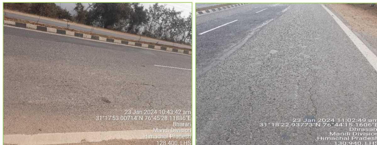
Figure: Alligator Cracks
