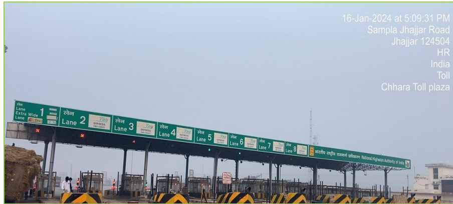
Figure 3-16: Over Head Lane Signal (OHLS).
