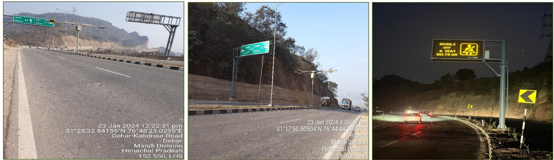
Figure 3-5: Overhead & Cantilever Gantry boards and VMS
